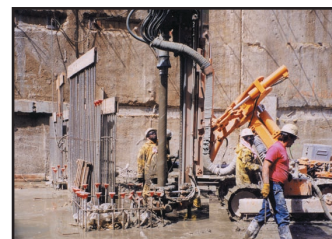
Fracturing/Regrouting
